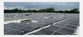
Working toward sustainability is a way of life at our Wabtec site in Piossasco, Italy. In 2022, the first phase of the solar project was constructed. The first panels are capable of producing 97 kilowatt hours (kWh) of power, equal to 5% of the Piossasco plant's annual electricity needs.
