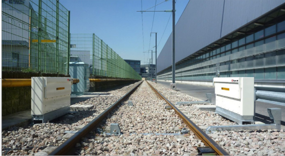
BEARING ACOUSTIC MONITOR
